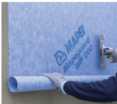
Pose de Mapeguard WP 200
