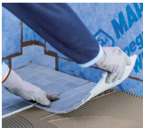
Pose de carrelage
